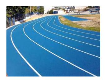
Synthetic outdoor system for running tracks in total thickness of 13.5mm.
