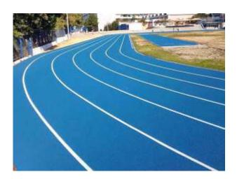
Synthetic outdoor system for running tracks in total thickness of 13.5mm.
