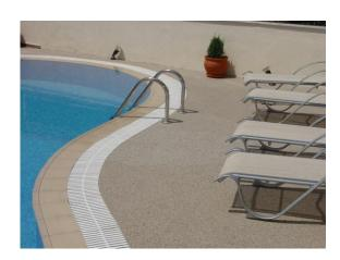
Consists of hard quartz aggregates and two-component polyurethane or epoxy or polyurethane resins.
