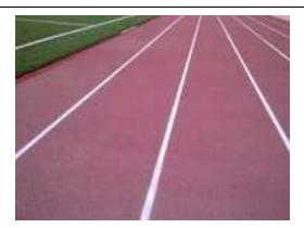
Innovative, new, synthetic outdoor economical system with a shock-pad for running tracks, in thickness of 13mm, or as outdoor system for refreshing old courts.
