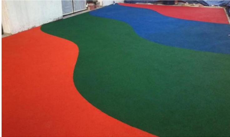
**Special formulated UV-resistant polyurethane**, two component, mat and glossy coating with additives with the parallel use of **EPDM 857 - epdm powder** and then **a top coat PU layer** to plasticize completely the flooring.
