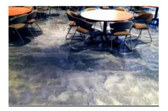
Epoxy-based, unique, self-leveling, three-component decorative flooring with special metallic pigments to create a brilliant, vivid, one-of-a-kind floor. Can be customized to produce unique, metallic-look, light-reflective floors.
