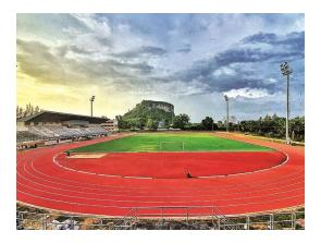
Synthetic outdoor system for running tracks in stadiums in total thickness of 15mm.
