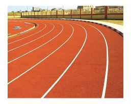
Synthetic outdoor system for running tracks in total thickness of 14.5mm.
