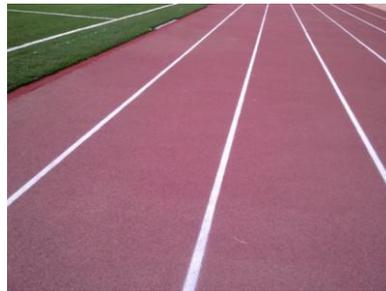
**Elastic, seamless ,flexible coloured flooring, ideal for jogging tracks.** It consists of a shock-pad base of 2 layers, first layer is a base layer of SBR granules (granulometry 2-5mm or 3-5mm) in thickness of 8mm up to 13mm and second layer a base of flexible, coloured epdm granules(0,5-1,5mm) in thickness of 5mm. Then follows a PU flexible pore filler coating in 2 layers and a sealing PU UV resistant aliphatic top layer in two crossing layers.
