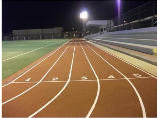
**Elastic, seamless, flexible coloured flooring, ideal for jogging tracks.** It consists of a base layer of SBR granules (granulometry 0.5-2mm) and then follows a PU flexible pore filler coating in 2 layers and a sealing PU UV resistant aliphatic top layer in two crossing layers.
