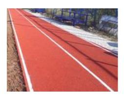
Elastic, seamless, flexible colored flooring, ideal for jogging tracks in total thickness of 18mm.
