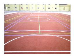
Outdoor highly flexible, acrylic system ideal for tennis, basketball, volleyball, handball, multipurpose courts, as well as any other outdoor sports court. Combination of prefabricated shock-pad and acrylic coating in average total thickness of 6 mm – 14mm.
